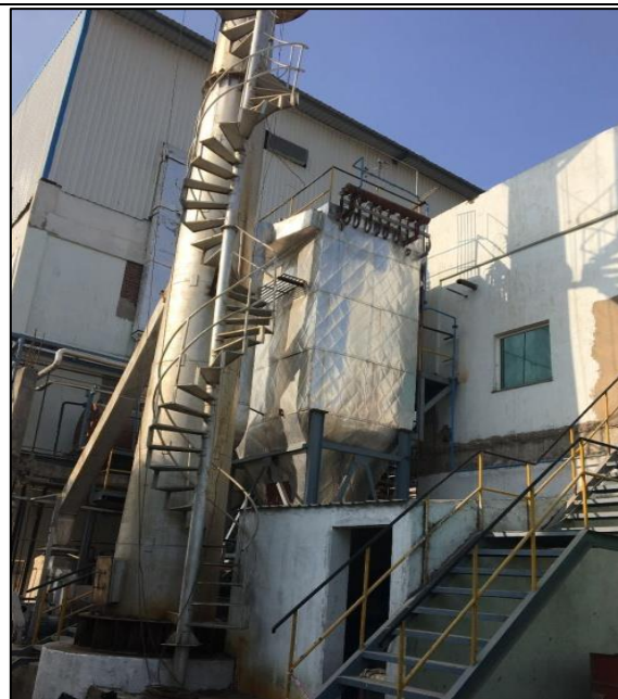
Bag filter attached with boiler stack
