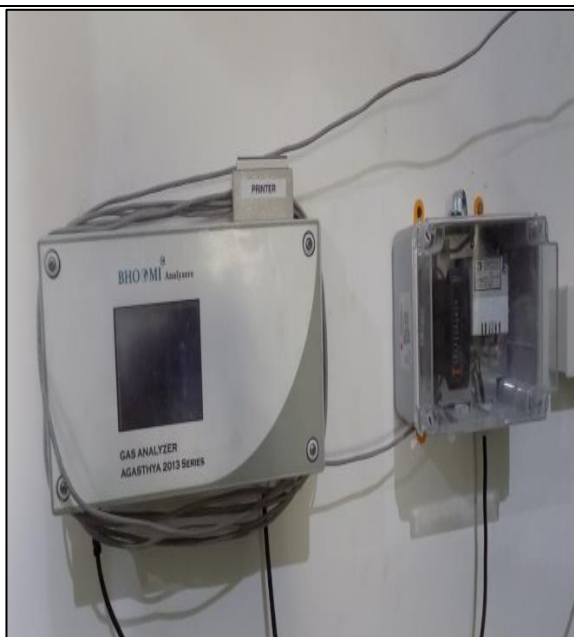
Boiler SPM Monitoring Panel
