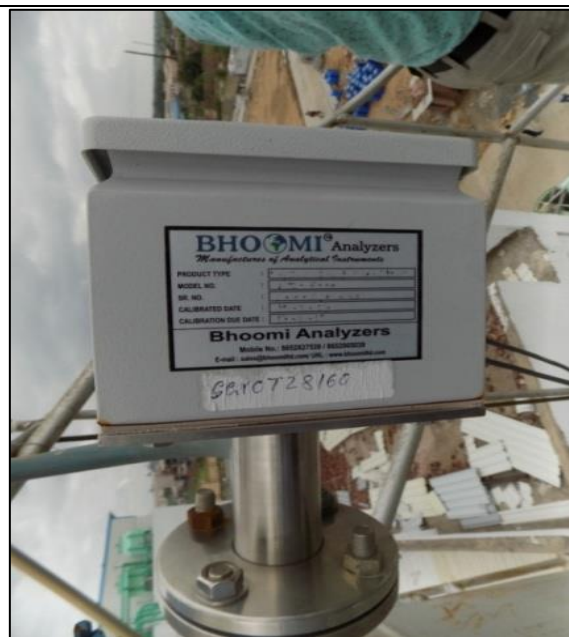
Boiler Stack Monitoring Sensor
