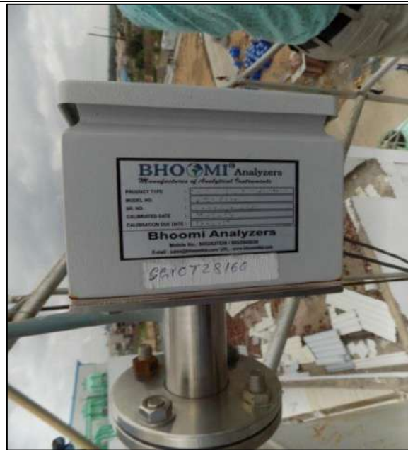
Boiler Stack Monitoring Sensor
